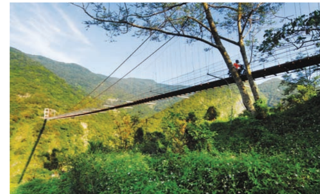
▼多納高吊橋 / Duona Suspension Bridge
